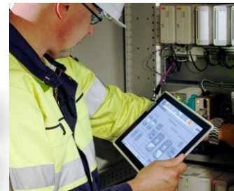
Mobile Panels [ABB]
